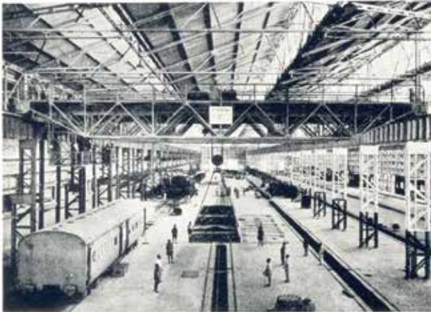
The main Assembly shop.
