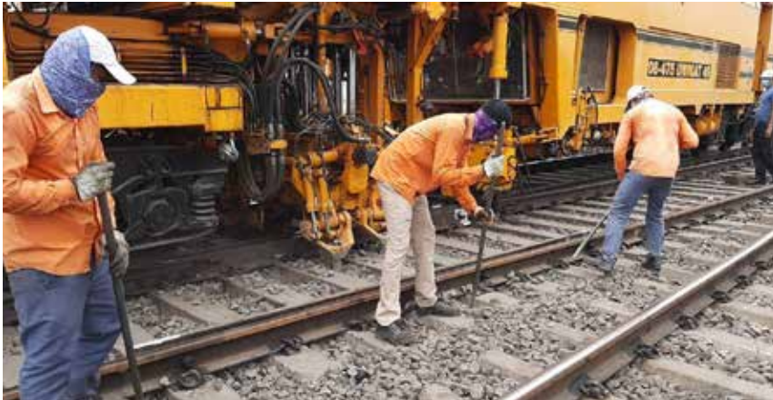
Relentless work done by the track maintainers.
