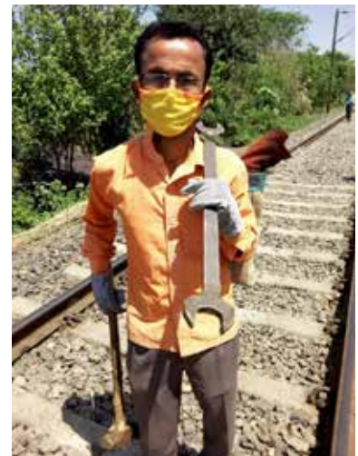
Our Trackman working on the track.
