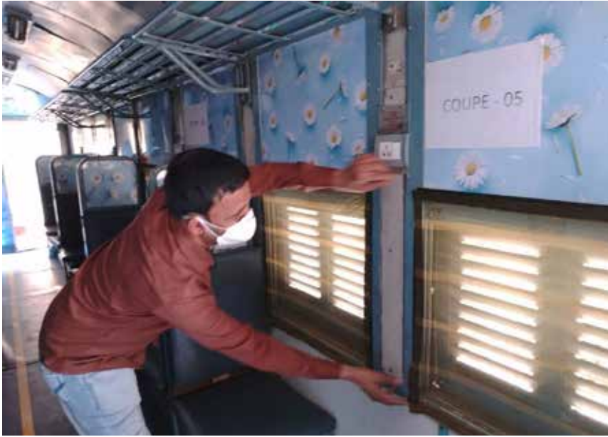
Work for conversion of passenger coaches into isolation coaches
